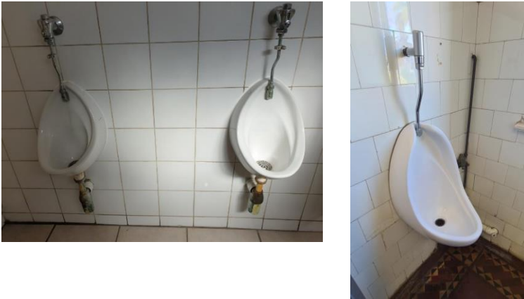
Figure 19: Examples of urinals with different flush mechanisms.
