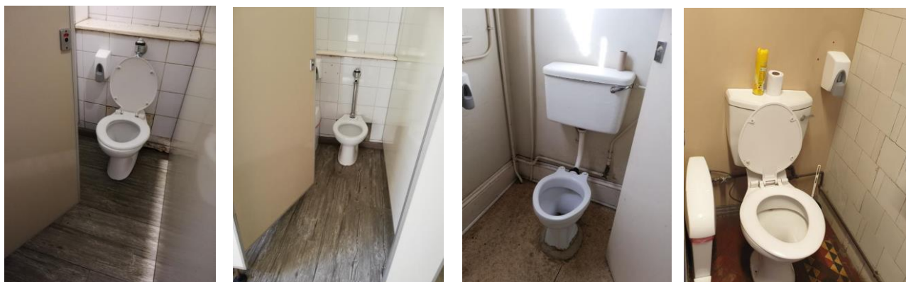
Figure 17: Examples of the various toilet types with different cistern sizes.
